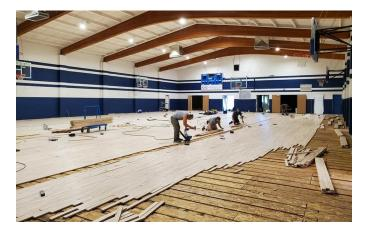
Work on the gym floor continues. As you can see in the above photo, the wood flooring has already begun to go in. However, they estimate that it will be roughly an additional 3 weeks following installation of the wood floors before the gym is able to be used.
